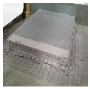
Figure 2: Un-bonded Screed, Training Mock-up, MPX Centre for Excellence
