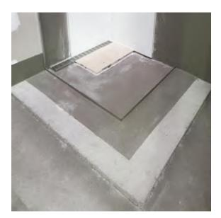
Figure 1: Bonded Screed, Training Mock-up, MPX Centre for Excellence
