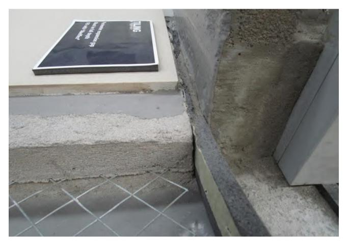
Figure 3: Full depth gap of 10mm through the tile bed, Training Mock-up, MPX Centre for Excellence
