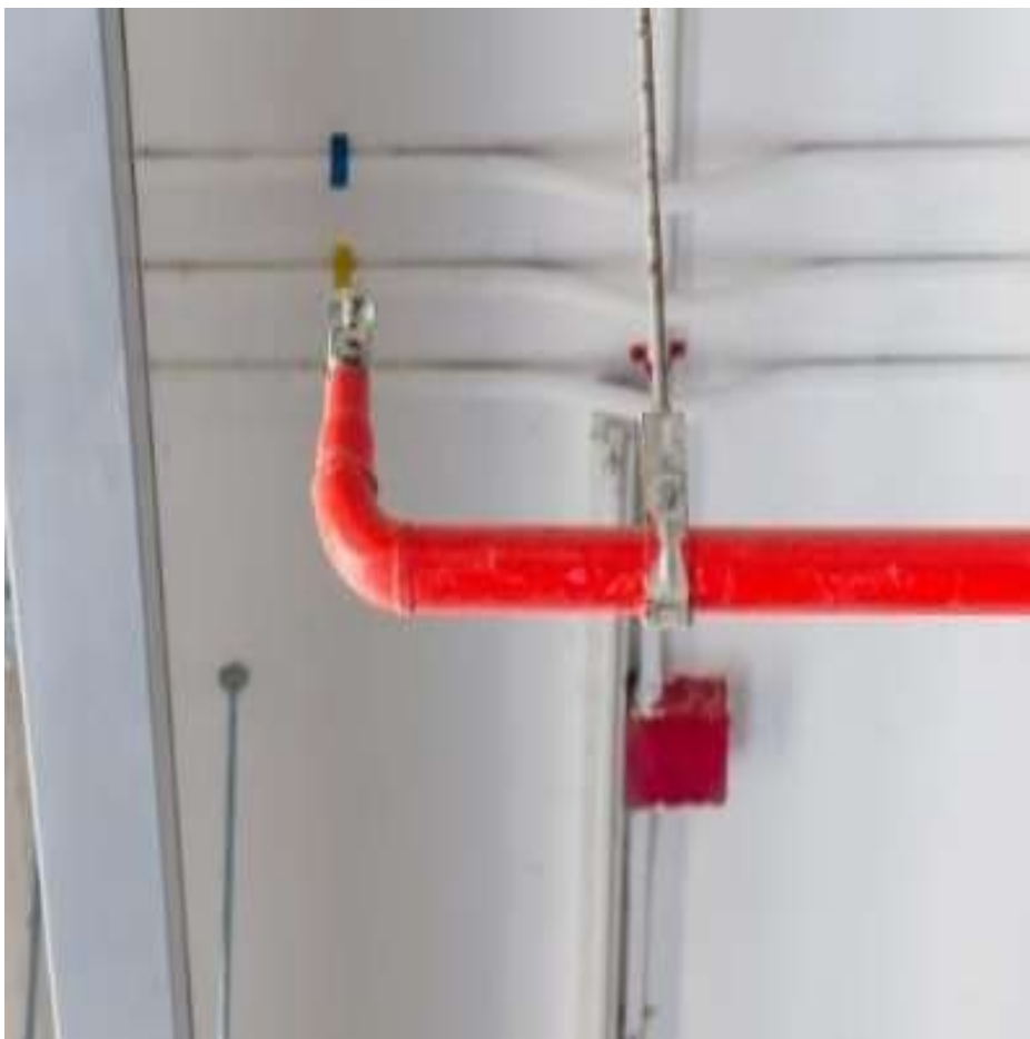
Figure 1: Range pipes supports over 500mm in length
