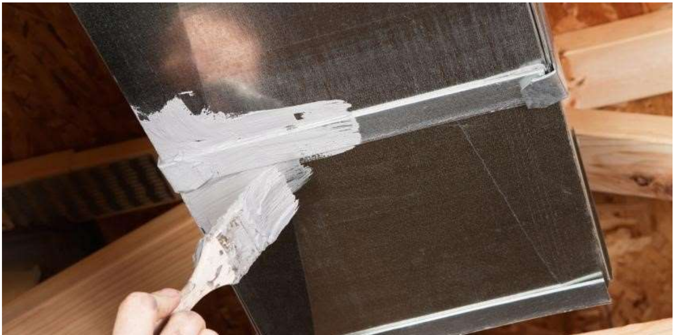
Figure 14: Sealing of duct joint corners and slide joints, source https://www.allbritten.com/air-duct-sealing
