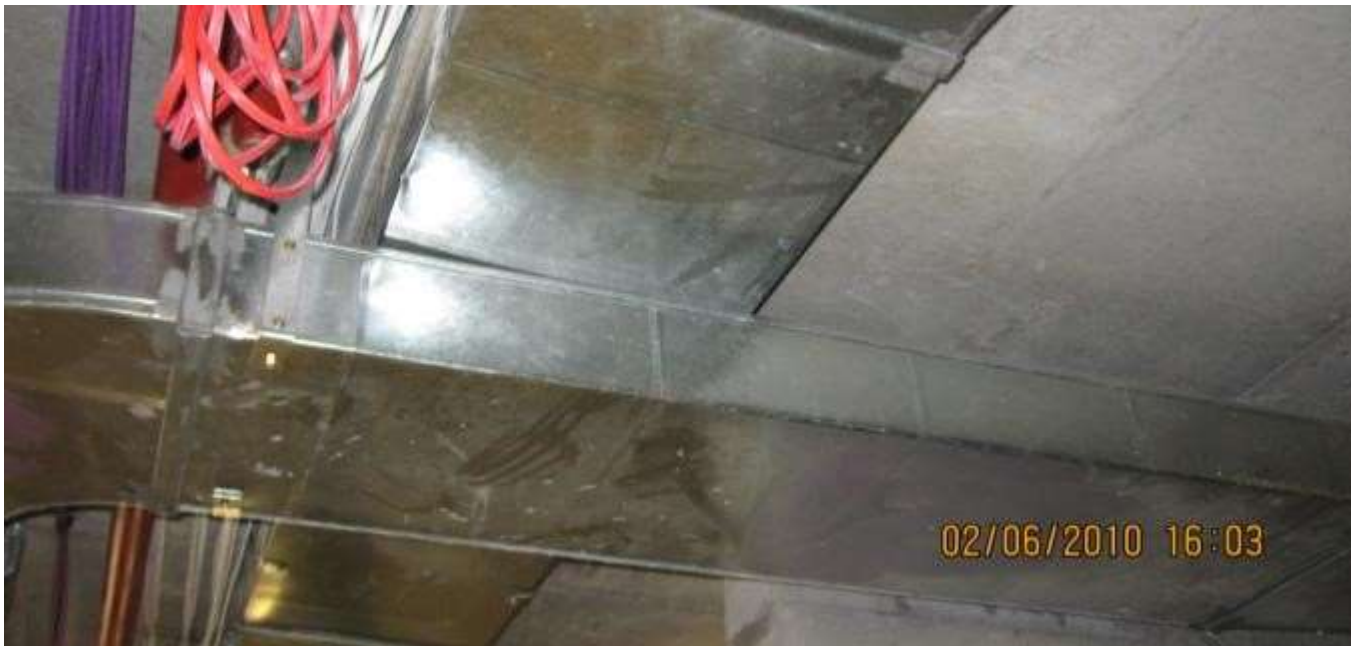
Figure 20: Ductwork in contact with other duct
