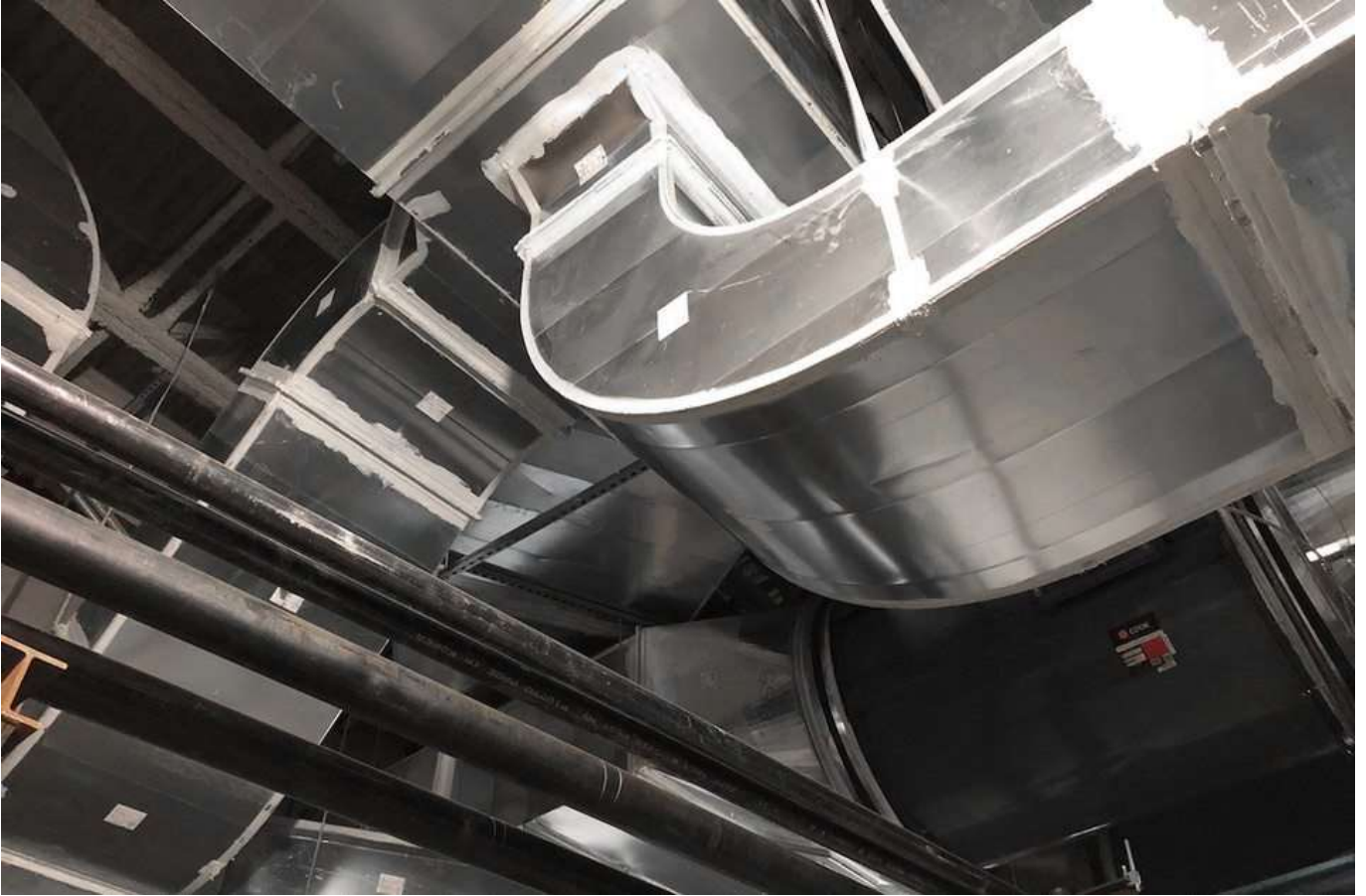
Figure 15: White mastic on all joints, Conklin Metal Industries
