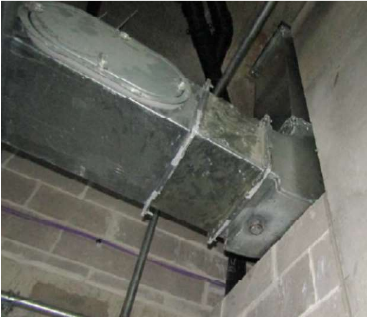
Figure 34: Kitchen exhaust systems – drain plug
