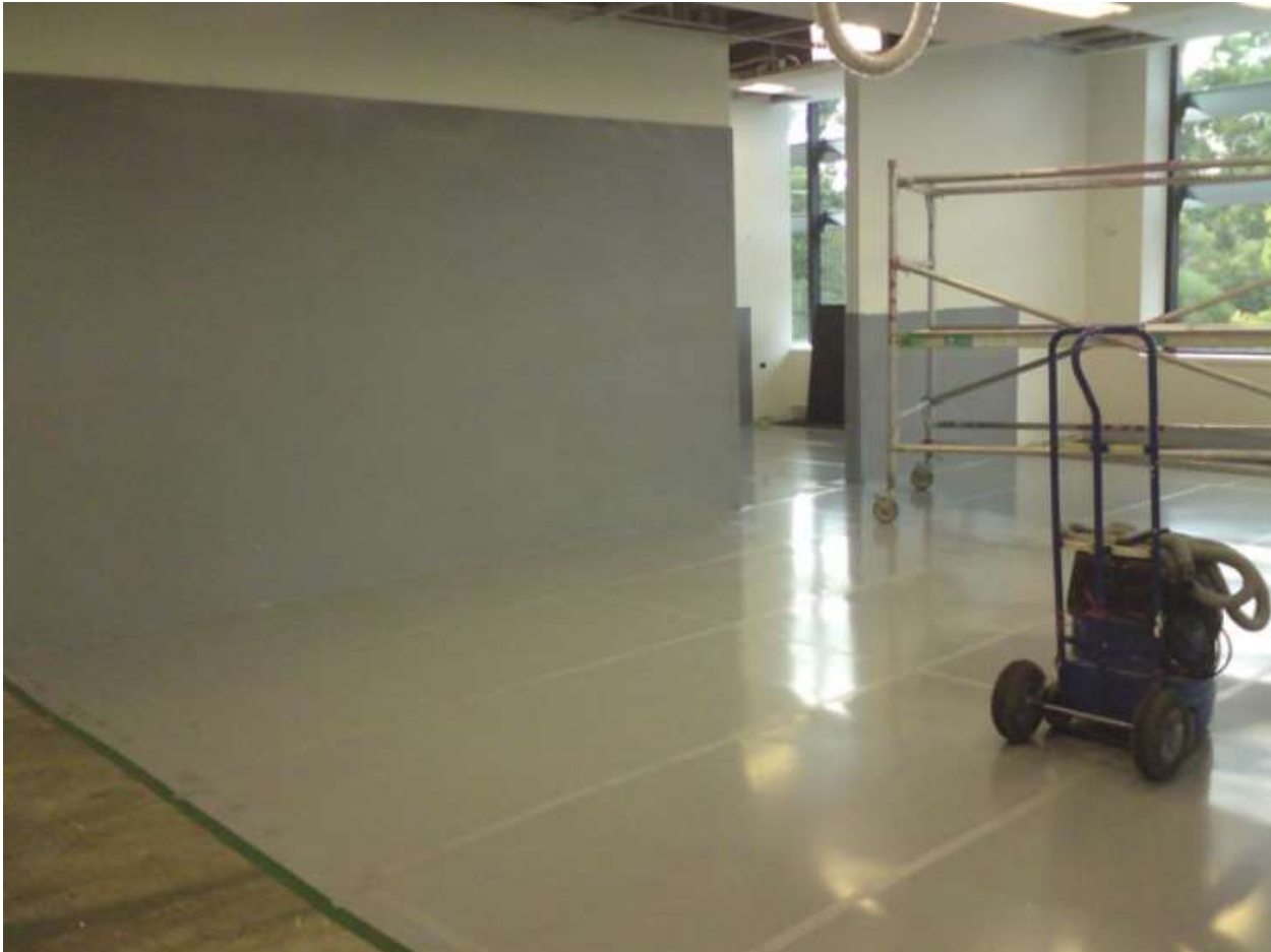
Figure 3: Carbon steel sheets being installed on walls & floors
