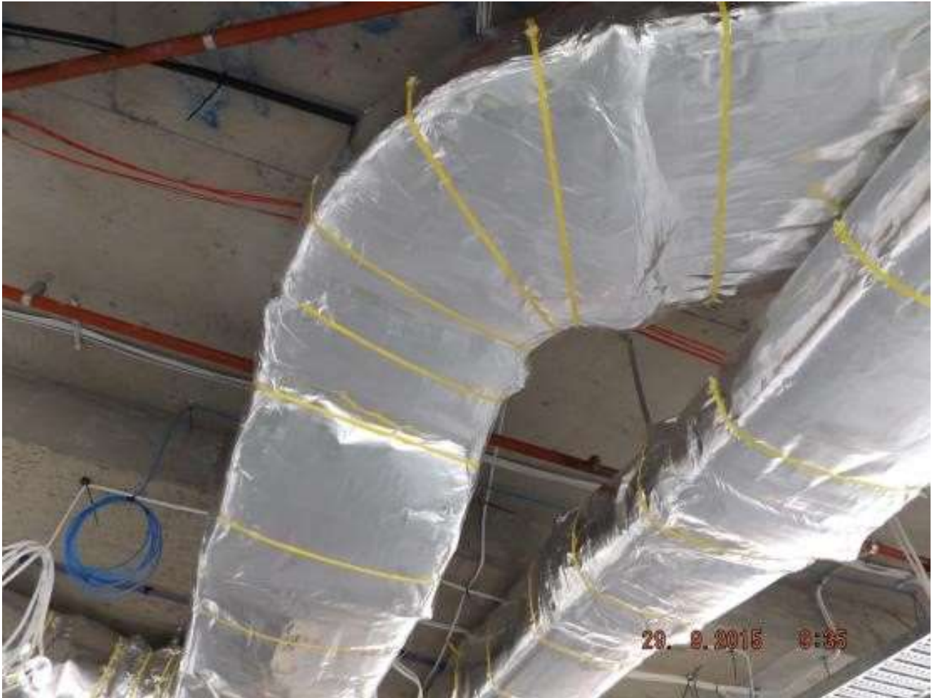
Figure 18: Ductwork insulation after hanging system is installed
