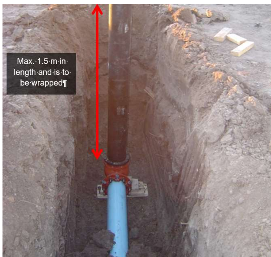
Figure 5: A hydrant riser connected to a plastic main
