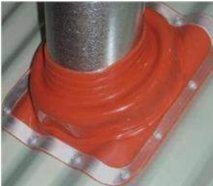
Figure 3: Red Dektites are used on flues and are heat resistant
