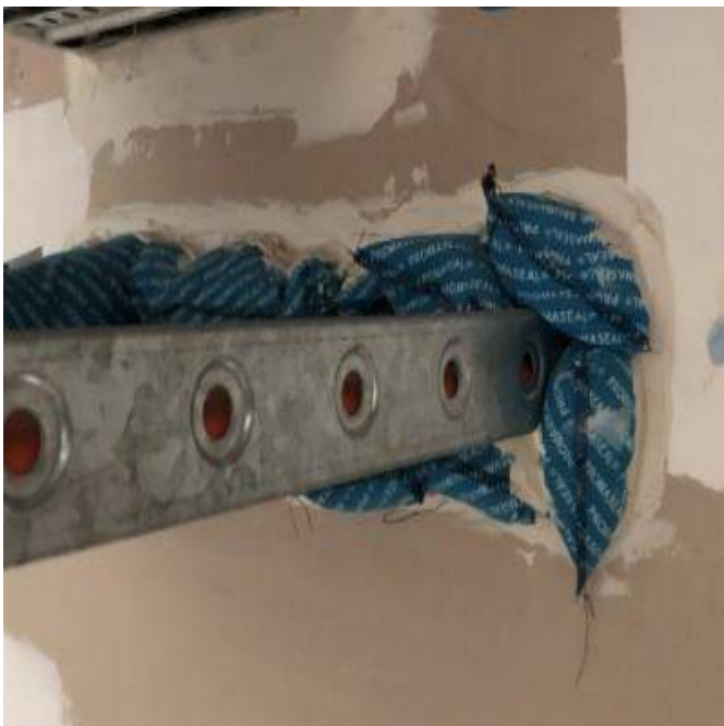
Figure 19 Cable Tray through Plasterboard
