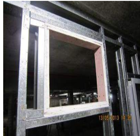
Figure 22: Framed and lined opening, MPX Training Mock-up
