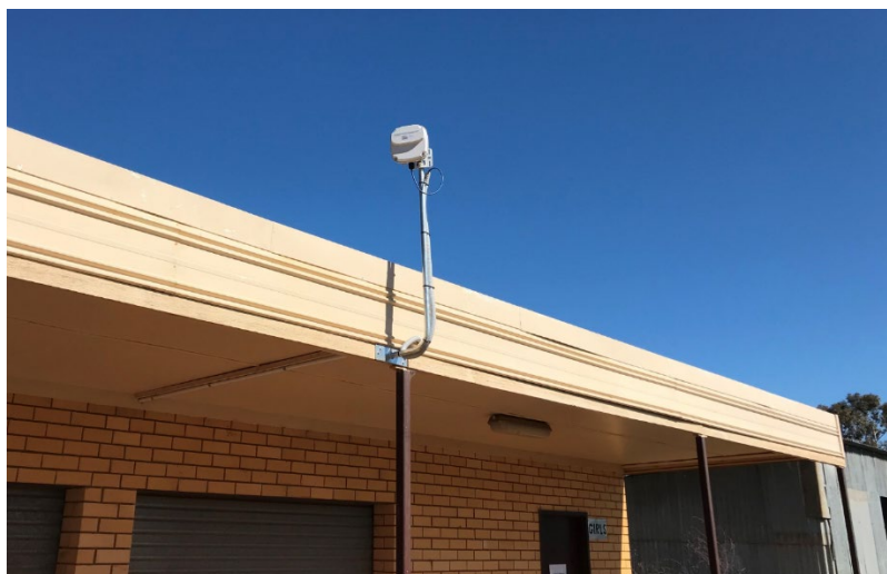
Figure 9 - Wireless bridge installation ref. 3 - BSP fitting and water proofing need to be followed as per instructions
