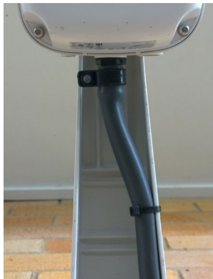
Figure 8 - External WAP installation ref. 2 (Note use of BSP fitting for cable ingress to WAP)
