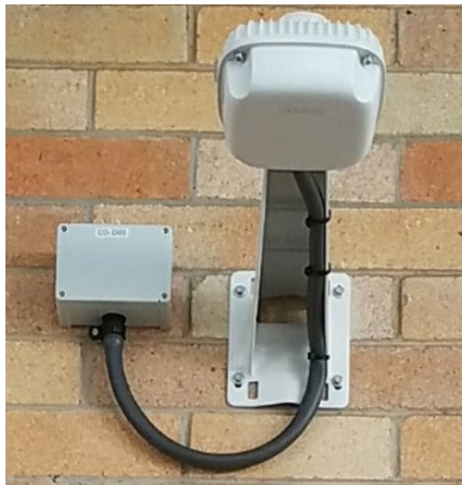
Figure 7 - External WAP installation ref. 1 (Note use of the waterproof cover)
