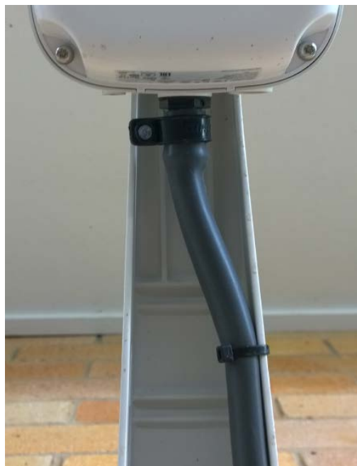
External WAP installation ref 2 (note use of BSP fitting for cable ingress to WAP)
